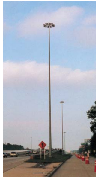
Light ring on top of pole is lowered by an RKI winch for maintenance.
